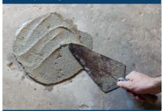
Substrates must comply with the specifications contained in the applicable and relevant standards for each country and area of application. Substrates must be sound and free of all traces of dust, loose or detached parts, varnish, wax, oil, rust and gypsum. New concrete substates should be fully cured. Repair any cracks present in the substrate with Adva-Repair Mortar.
