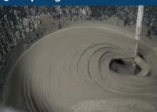
Pour a 20 kg bag of Adva-Level T315 into a bucket containing approximately 5 liters of clean water and mix with a low-speed electric mixer to obtain a homogeneous, self-levelling lump free mix. Keep the mix for 23-minutes as slackening time then the mix should be restirred prior to use. The amount of Adva-Level T315 mixed at any time must be used within 2030-minutes (at a temperature of +23°C).
